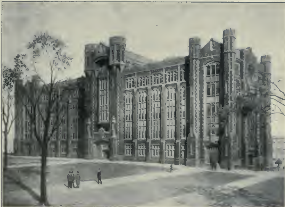
Ottawa Examining Warehouse—Stone supplied by Wallace Sandstone Quarries Company.
